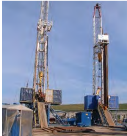
Figure 4. View of drilling rigs in Lagoszew, Poland.
