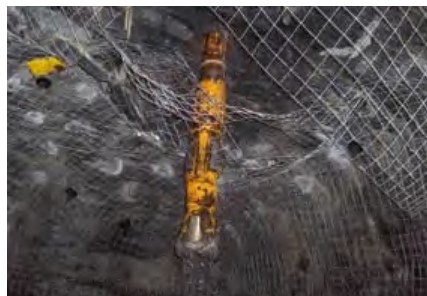
Figure 6. Break-through with RVDS in Rouyn, Canada.
