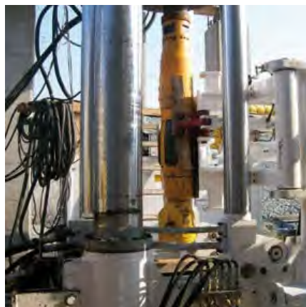
Figure 5. Installation of the RVDS in RBM Robbins 85R.
